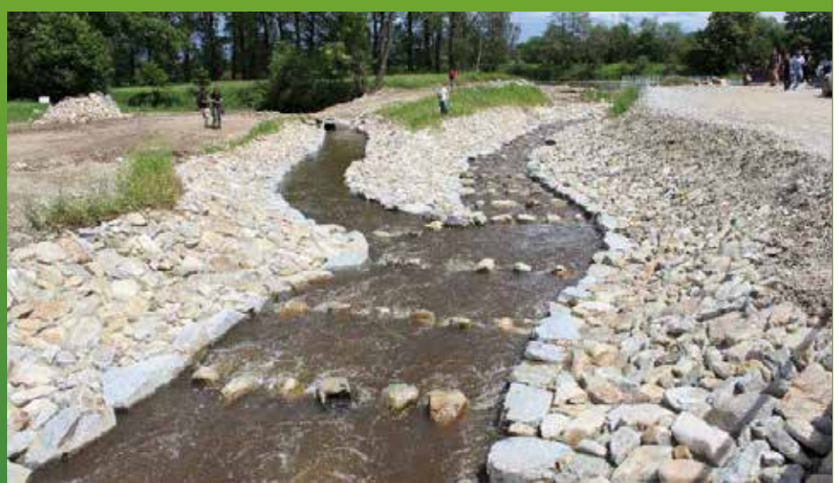
Bypass with the baffle fishway in the River Vltava (Planá)
