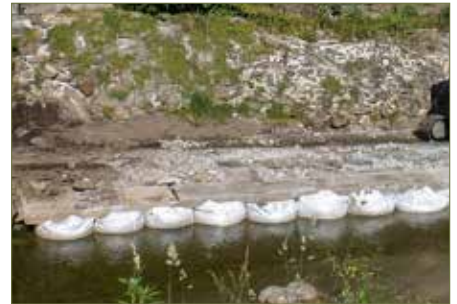
Fig. 4: Construction road on big bags
