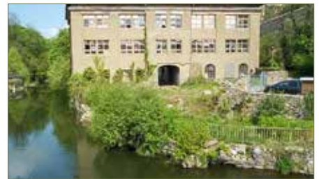
Fig. 6: Industrial wasteland before
