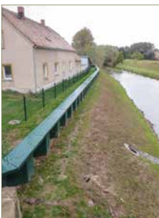
Fig. 5: Flood protection in Halbendorf, left free-standing sheet pile wall, center covered sheet pile wall, right new flood protection mill Halbendorf
