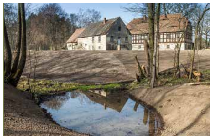
Fig. 5: Flood protection in Halbendorf, left free-standing sheet pile wall, center covered sheet pile wall, right new flood protection mill Halbendorf
