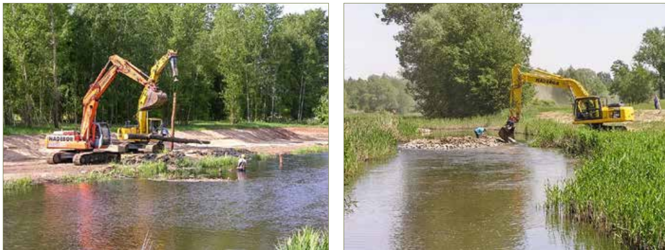
Fig. 1: Measures to improve the structural diversity in the Spree. Left – Installation of wooden groynes, right – construction of a river island
