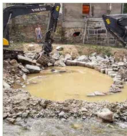
Fig. 10: Construction of the screw groyne
