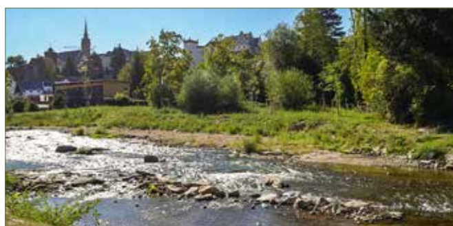
Fig. 11: Deconstruction weir 3 – above before – below after
