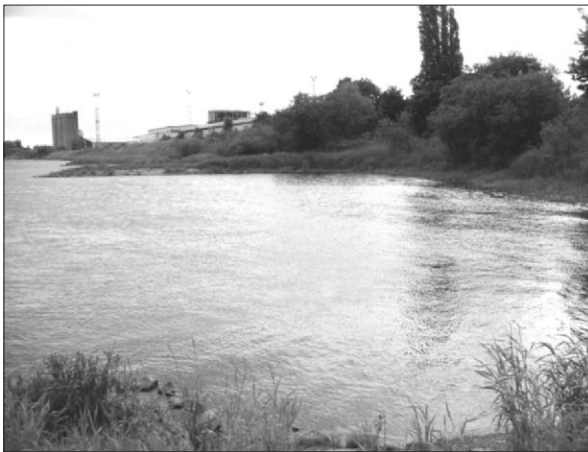
Fig. 1: Groyne field Fahlberg, near Magdeburg.
