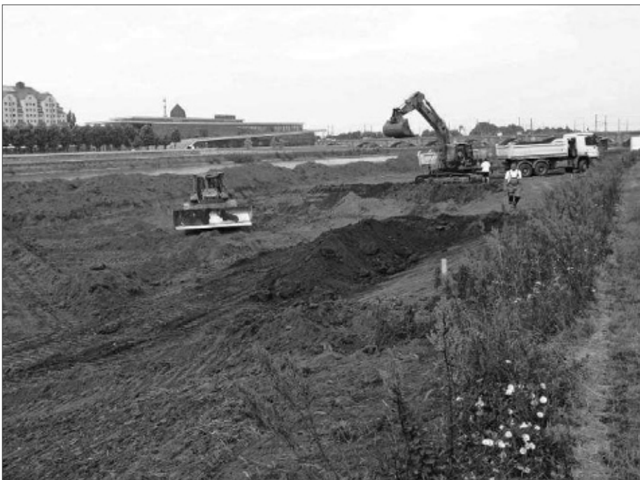
Abb. 2. Foreland excavations on the Dresden Neustadt side. Photo by Environmental Office
