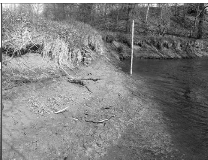
Pic. 7: Erosion of the banks of the Kössein
